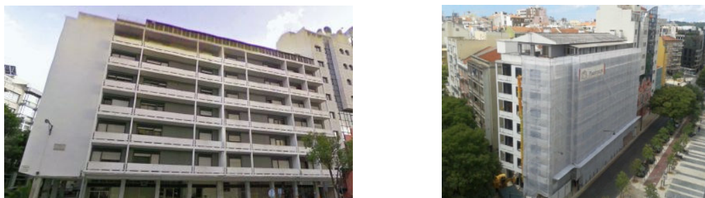
Figure 1. Building façade and a general view.
